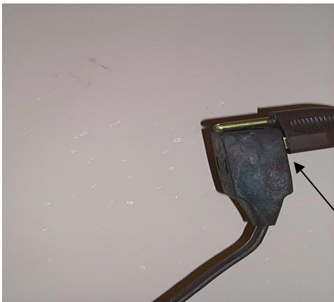
Figure 2 Three prong plug into a two-wire extension cord
